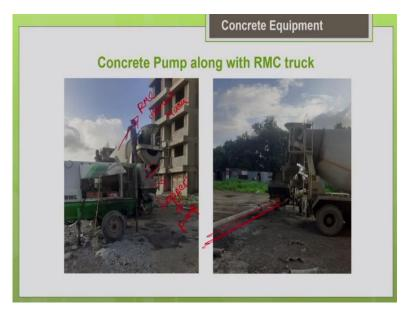
So, this picture shows you the concrete pump along with the RMC transit mixer. So, you can see this is the RMC transit mixer. This is your RMC transit mixer. So, it is delivering the concrete through the chute. The transit mixer will have a chute. With the help of the chute it is delivering the concrete into the hopper of the pump. So, from the pump, as we discussed based upon the piston action, the concrete will be delivered into the delivery pipelines.
